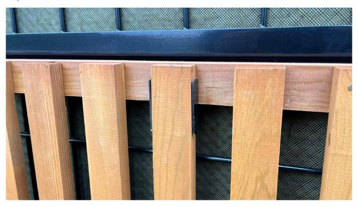
**Step 5**Fix the position in such a way that its side edges match the side edges of the metal panel's flat bars.
